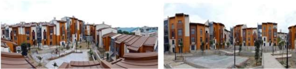
Figure 2: New building in Sulukule after urban transformation ( http://www.fatih.bel.tr/icerik/1155 )
